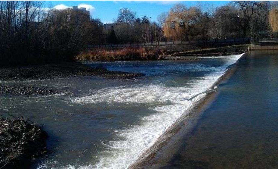
Partial demolition of the San Marcos weir (Bernesga river, León-Spain)
