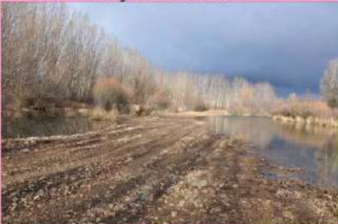
Works recently completed
