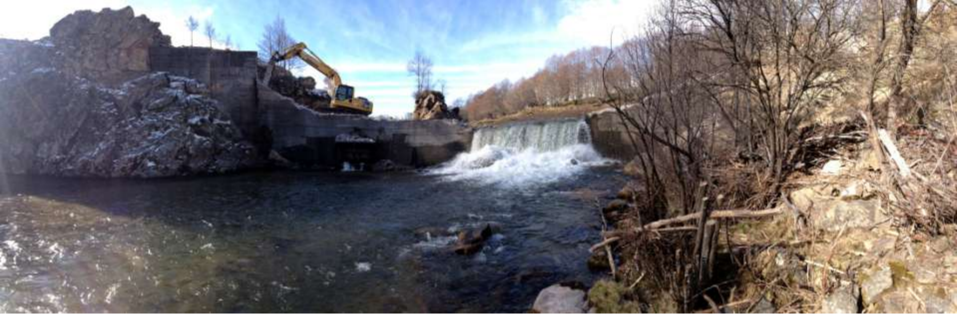
Demolition of the Umbrías dam (Aravalle river, Ávila-Spain)
