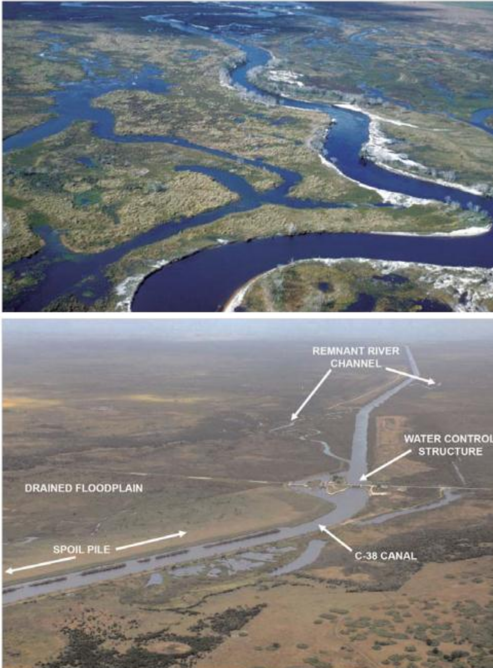
Figure 12: Photographs of the Kissimmee River prior to channelization and after channelization
