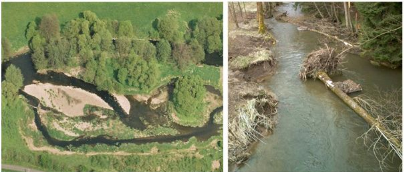
Figure 1: Two typical restoration projects included in the database, focusing on channel planform (left, © A. Lorenz) and instream channel features (right, © W. Klein).
