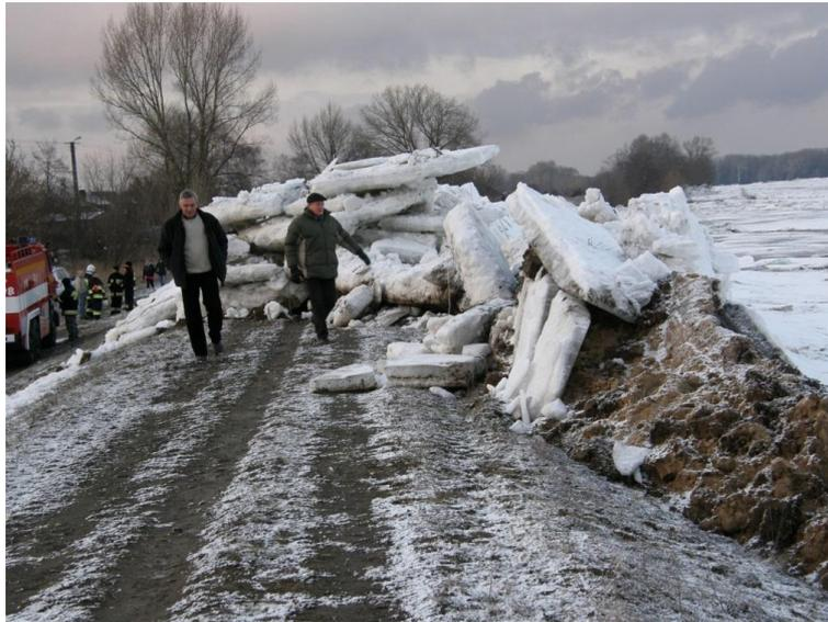
Figure 6.16. Ice-jam on the Vistula near Plock (04.03.2010) – damaged embankment at km 597
