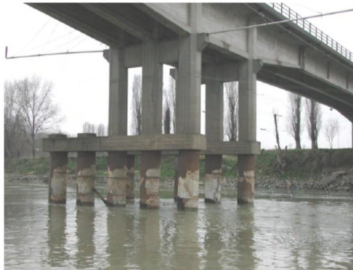
Figure 3.11 Bridge piles on the Po River (Boretto): evidence of channel incision. Extracted from Bertolo et al. 2009.
