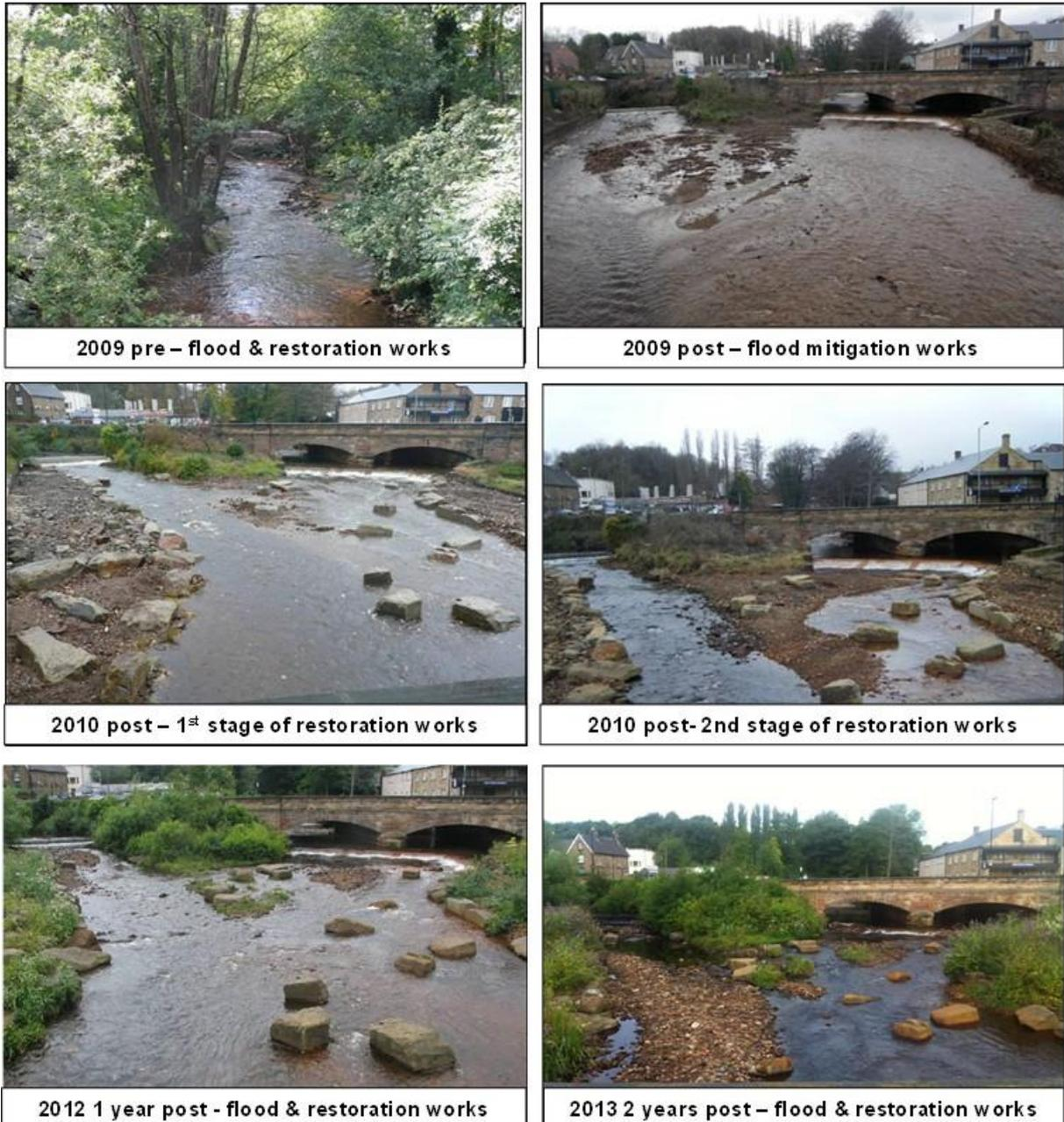
**Figure A-2: Point photography at Malin Bridge to show the morphological changes made to the River Rivelin (left) and Loxley (right) post-flood works in 2009 and post-restoration works in 2010 and 2011.**
