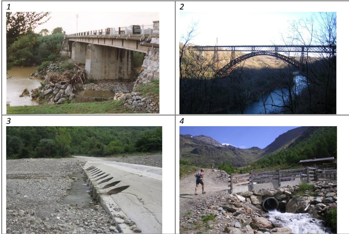
Figure A3. 47 Crossing structures. (1) Bridge with interference on fluvial dynamics; (2) crossing structure unrelated to the fluvial corridor; (3) ford with culverts; (4) culvert.
