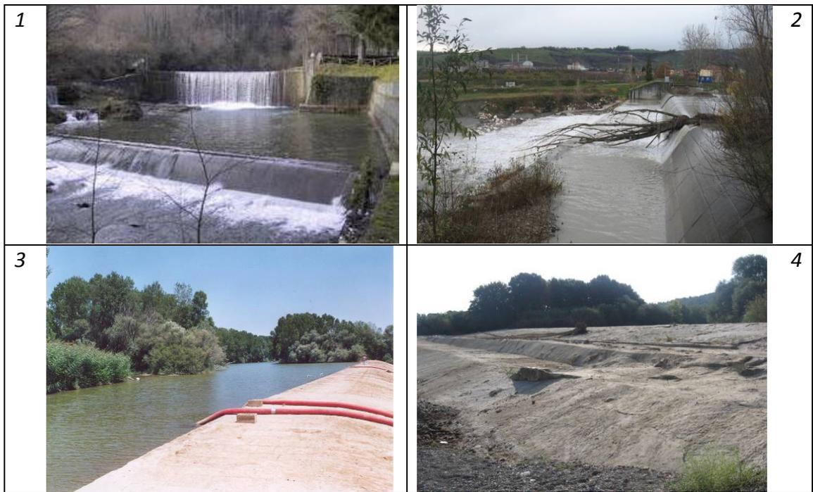
Figure A3. 40 Transversal structures of alteration of sediment discharges in hilly and lowland areas.
