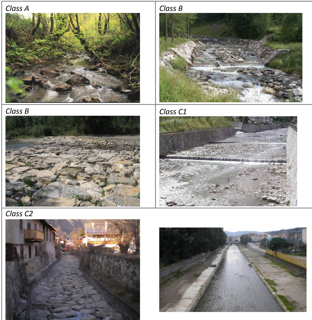
Figure A3. 58 Other bed stabilization structures and revetments.
